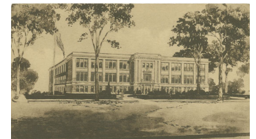
Morristown High School in process of construction
